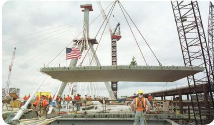
Construction of the Zakim Bunker Hill Bridge, Boston, Massachusetts
